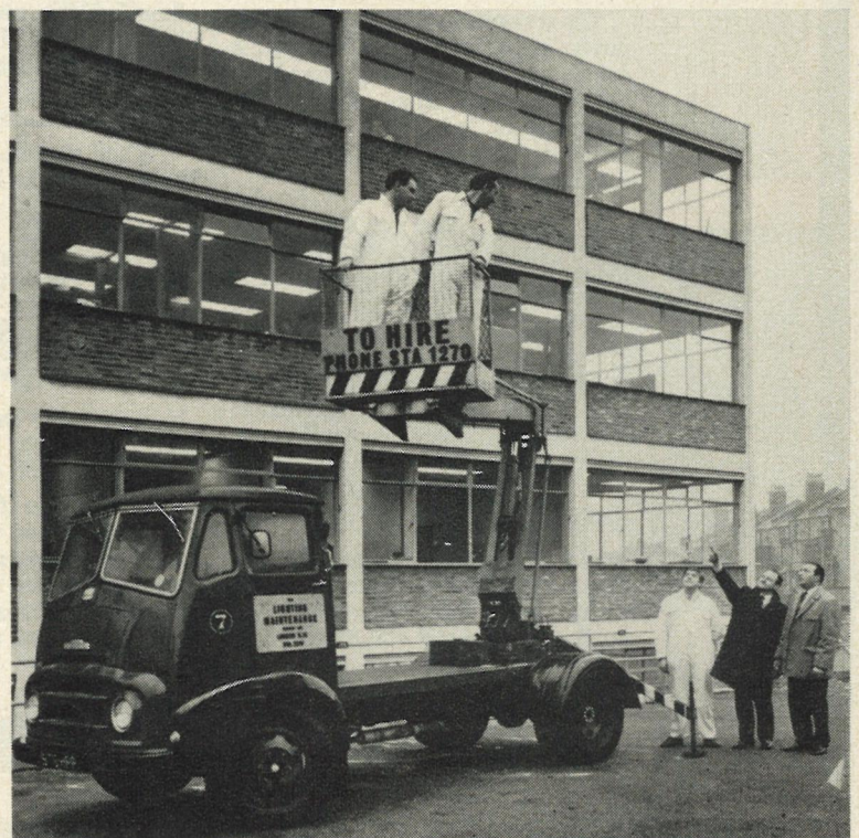
Simons arm vehicle for high level maintenance
